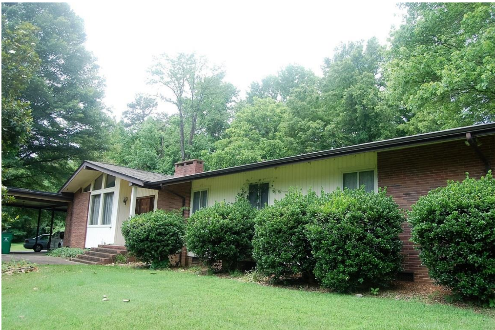
Triston G. and Barbara Stegall House, Façade, Looking Southwest.
