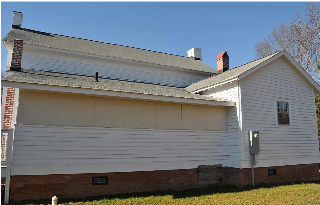
Harkey-McEwen-Moore House, After Relocation, 2016, East (Rear) Elevation, Looking West.
