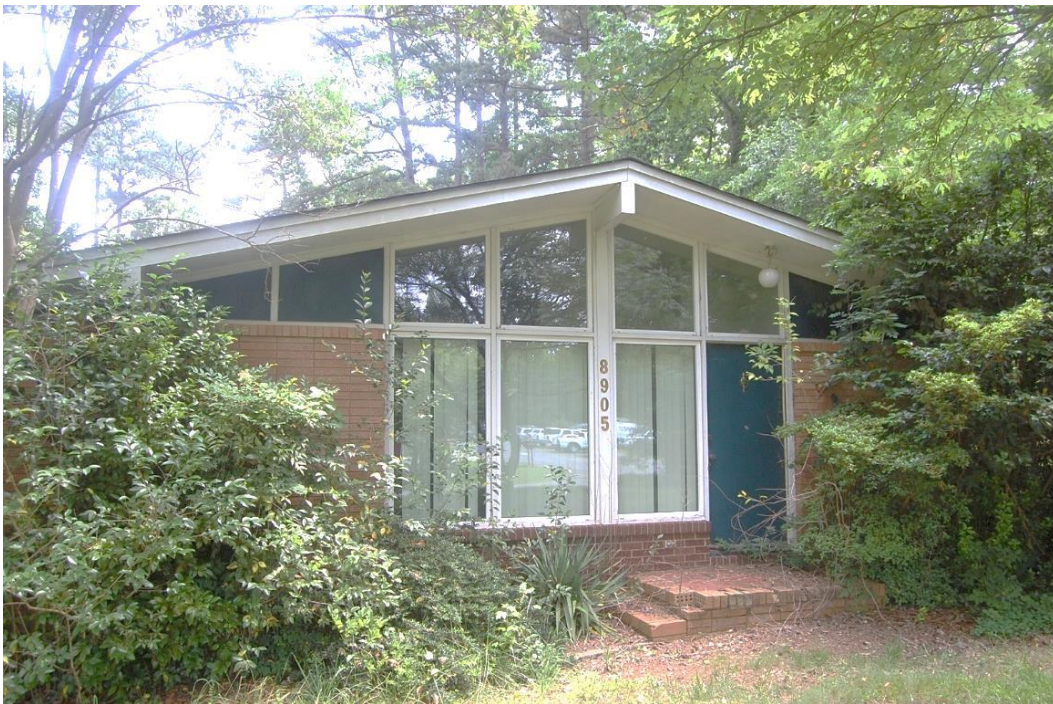
Layton E. and Margie Duncan House, Façade, Looking East.
