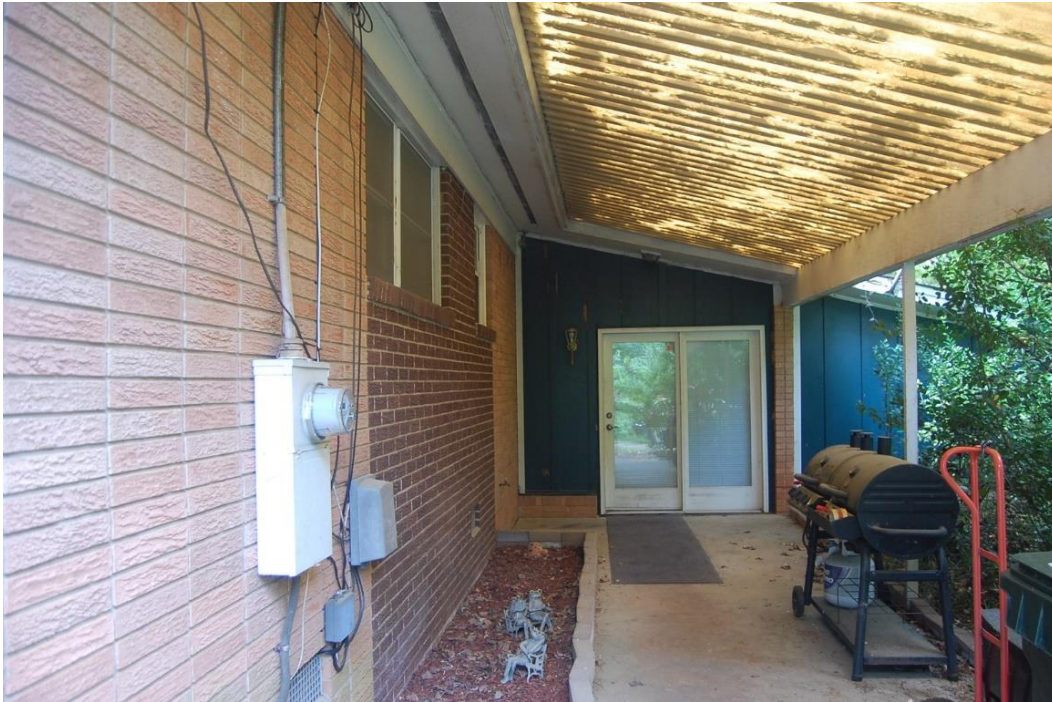
Layton E. and Margie Duncan House, Rear (East) Elevation, Rear Entrance, Walkway, and 4Garage, Looking West.
