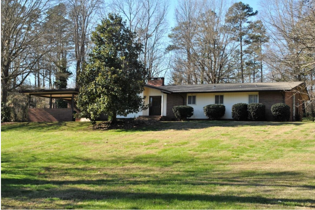
Triston G. and Barbara Stegall House, Overall View, Looking West.
