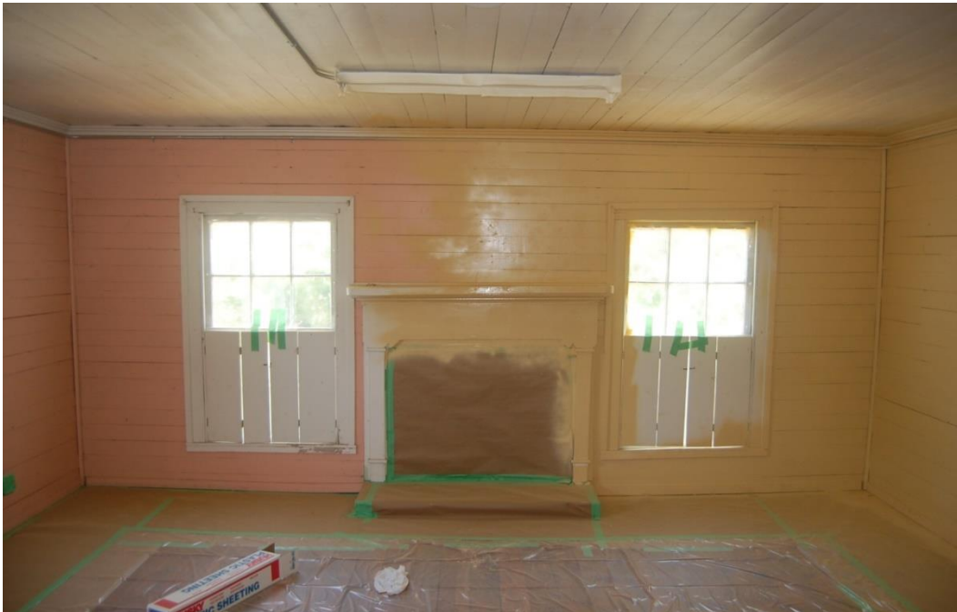
Harkey-McEwen-Moore House, After Relocation, 2016, Interior, North Bedroom.
