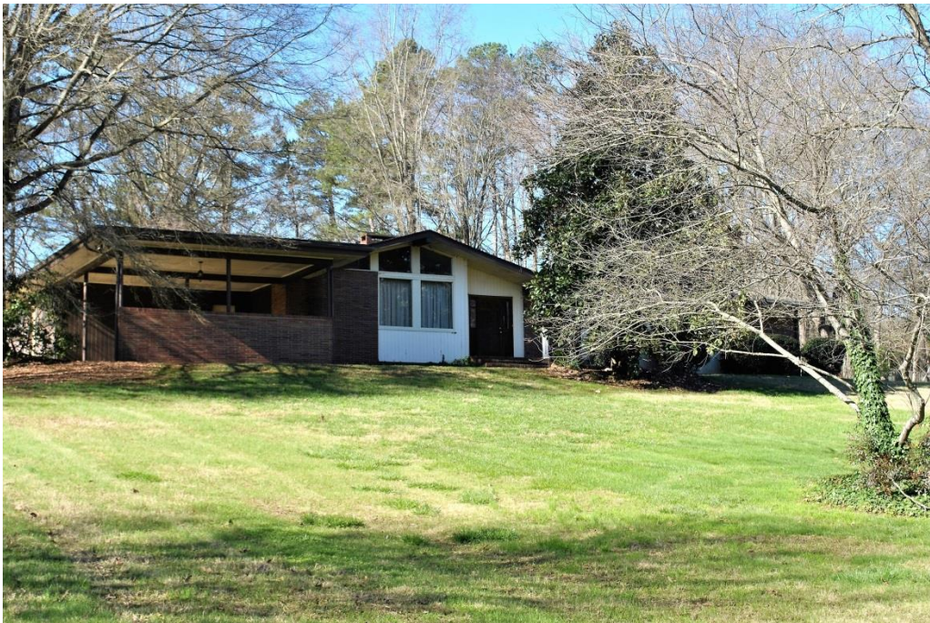
Triston G. and Barbara Stegall House, Overall View, Looking Northwest.
