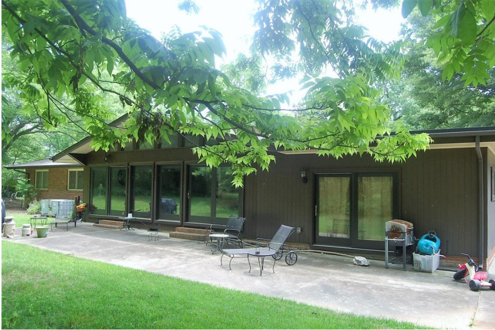
Triston G. and Barbara Stegall House, Rear (West) Elevation, Looking Northeast.
