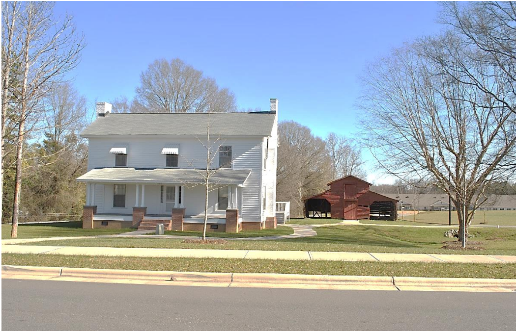
Harkey-McEwen-Moore House, After Relocation, 2016, Looking East (Modern Healthcare Facility in Background).
