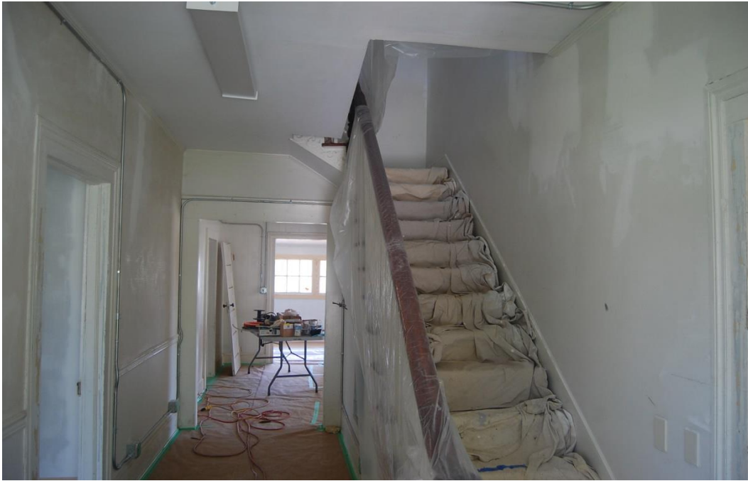
Harkey-McEwen-Moore House, After Relocation, 2016, Interior, Center Hall and Staircase.
