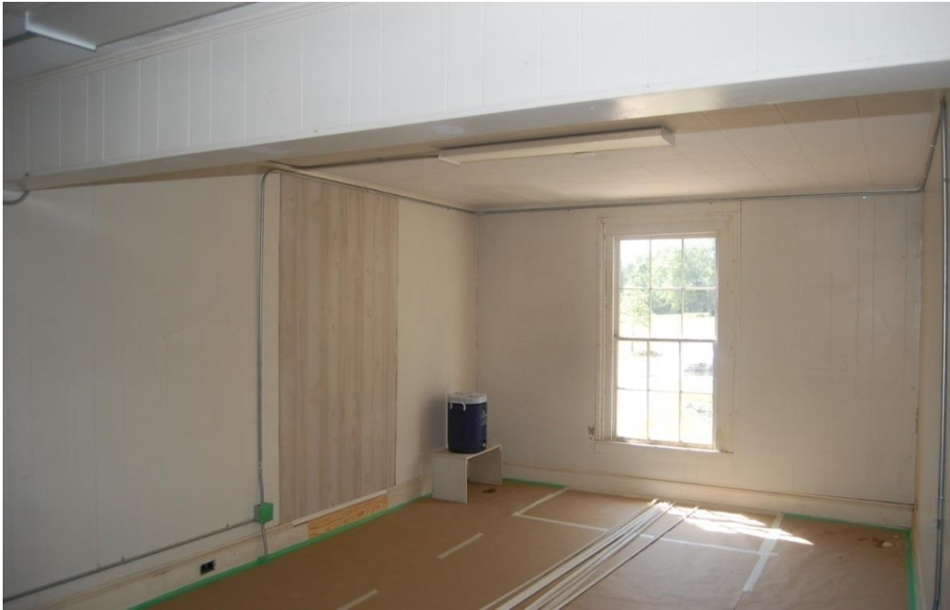
Harkey-McEwen-Moore House, After Relocation, 2016, Interior, Rear Shed.
