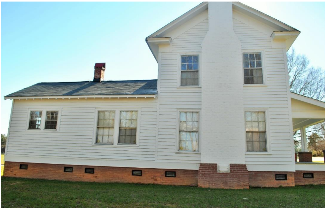
Harkey-McEwen-Moore House, After Relocation, 2016, North Elevation, Looking South.
