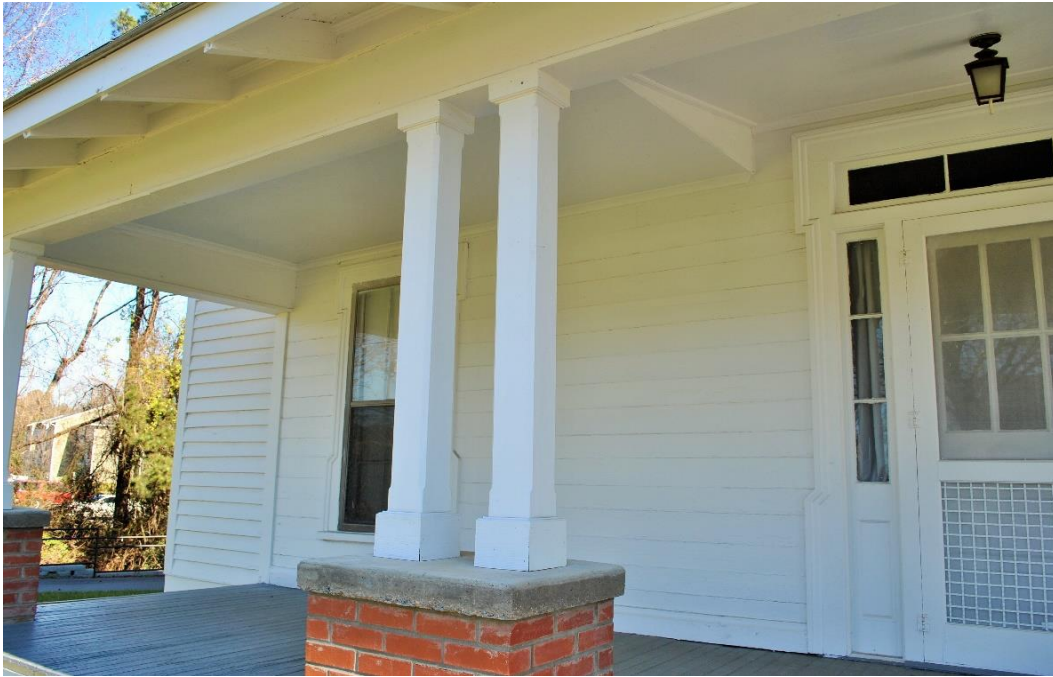
Harkey-McEwen-Moore House, After Relocation, 2016, Porch Posts, Looking Northeast.
